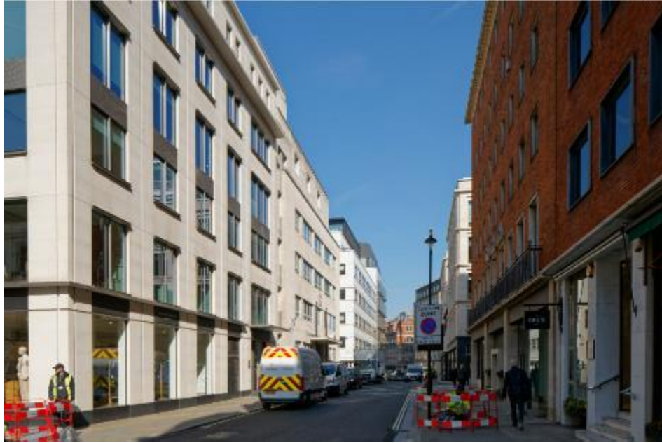
Existing view from Savile Row, looking north-west:
