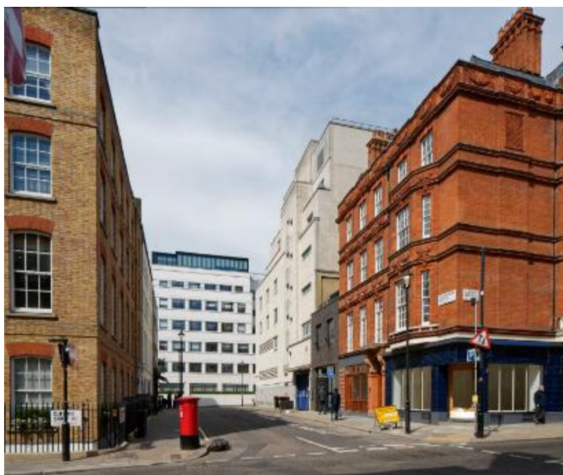
Existing view from Clifford Street, looking north-west:
